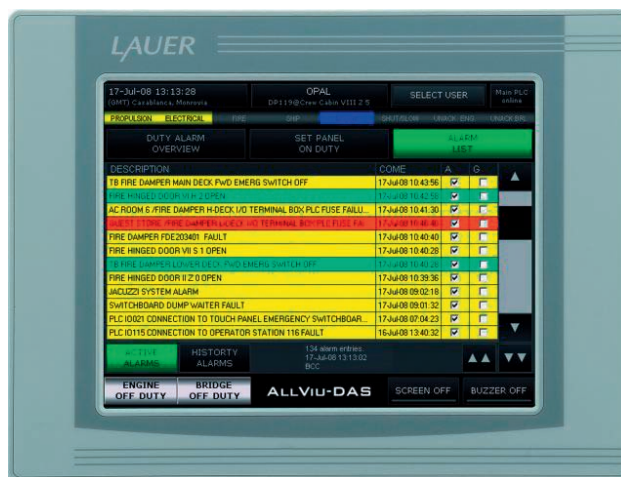
The 8.4” LAUER Nautic-PC is used as a Duty Alarm Panel in the Chief Engineer’s cabin
