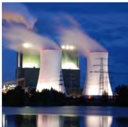
■ Block unit power plant
