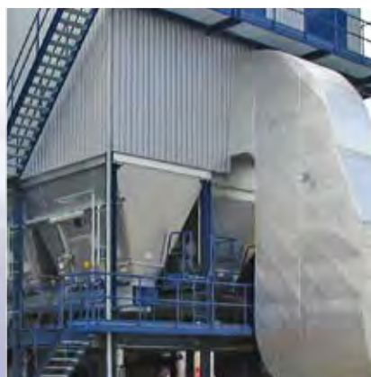
■ Dust filter cleaning
